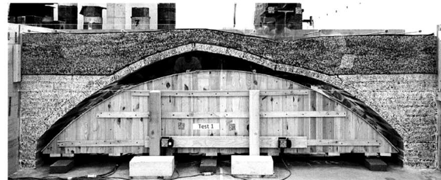
Fig. 8. Crack pattern and failure mode of UNR specimen.
